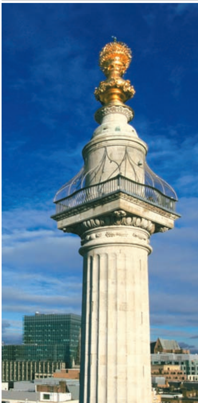
LONDON'S MONUMENT statue was re-opened yesterday after an 18-month restoration project. The 202-foot structure was declared a "symbol of hope" by surveyor Peter Bennett, who was in charge of the £4.5m restoration. A viewing platform has been installed, along with enhanced lighting. The statue, designed by Christopher Wren, was erected as a memorial to the 1666 Great Fire of London. Picture: SUE SALTON PHOTOGRAPHY
